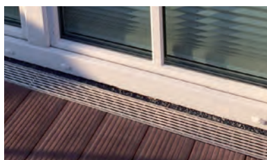
Open channel without a connection: terrace with the ACO Self® Highline
