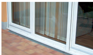
Closed channel with a connection to the soakaway system: façade with the ACO Self® Hexaline
