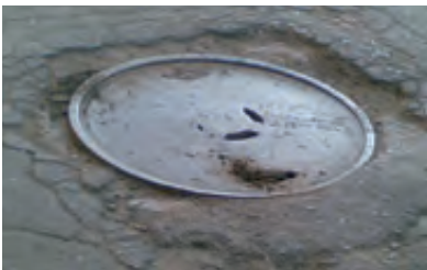
Damaged road surface due to low frame height
